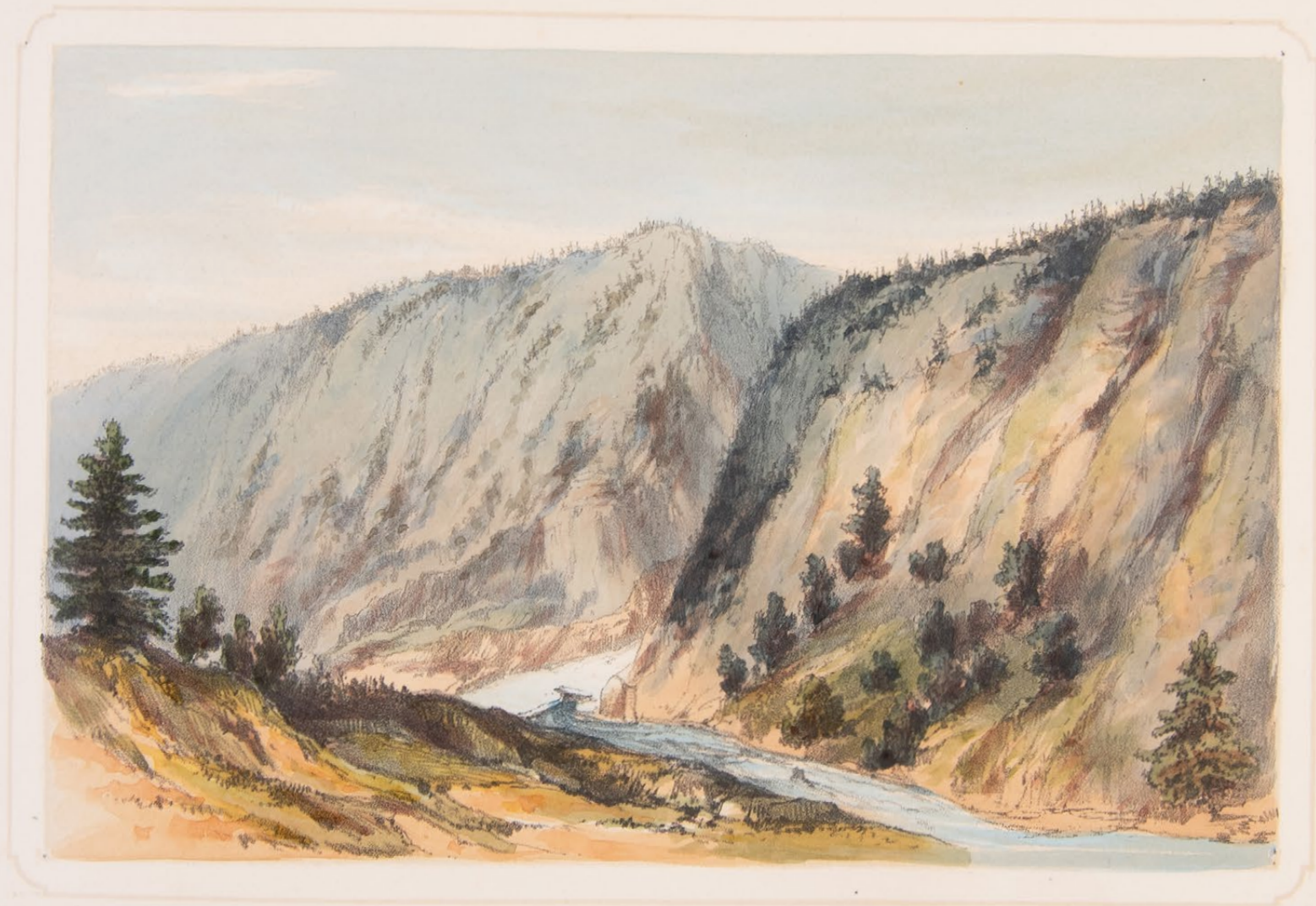
UPPER VIEW OF THE SNOW BRIDGE.
